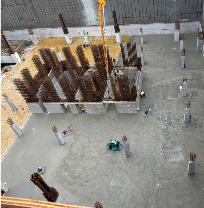
November 3, 2025: Preparation for P5 formwork progressing.
