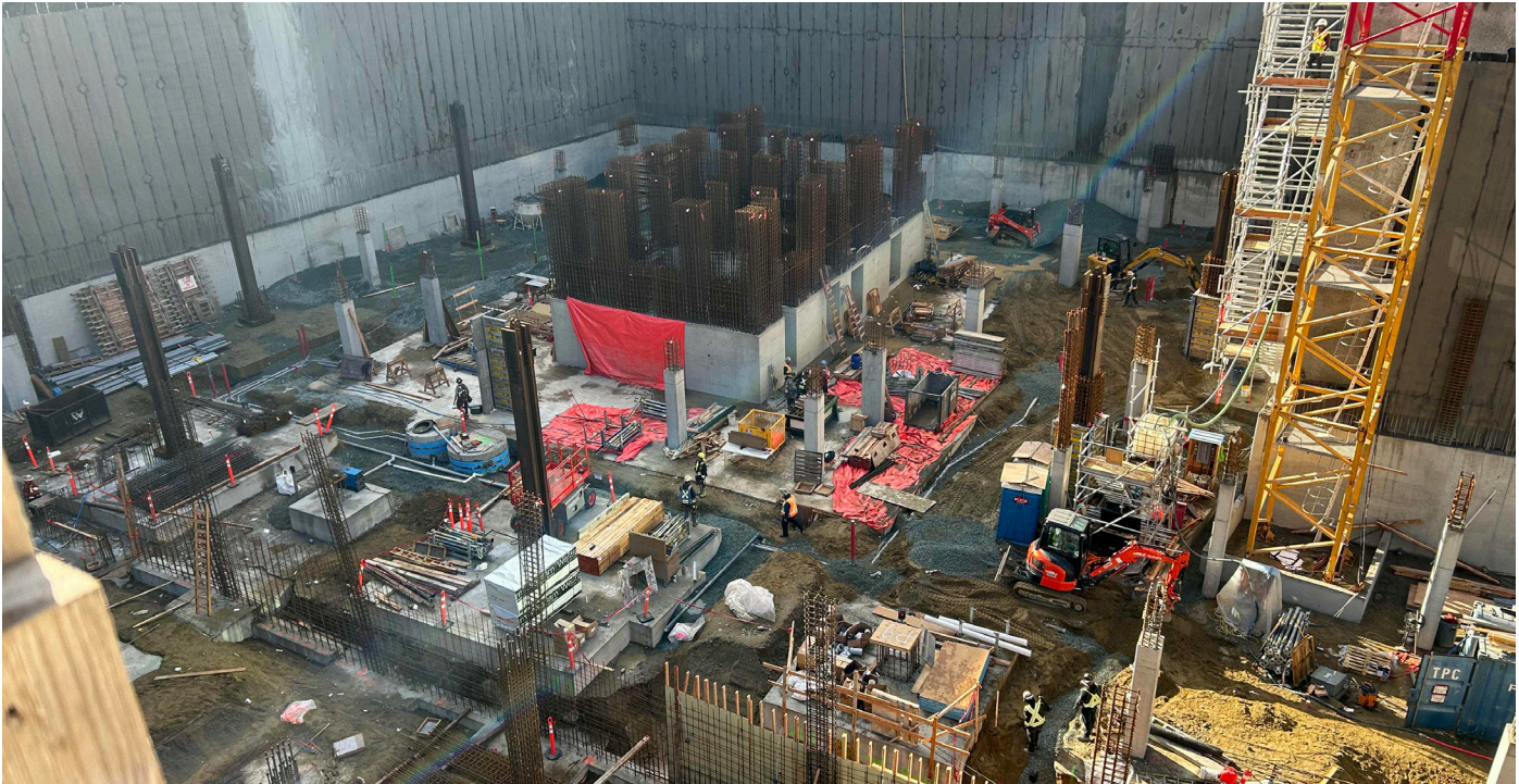
October 17, 2025: Progress on vertical concrete work ongoing.
