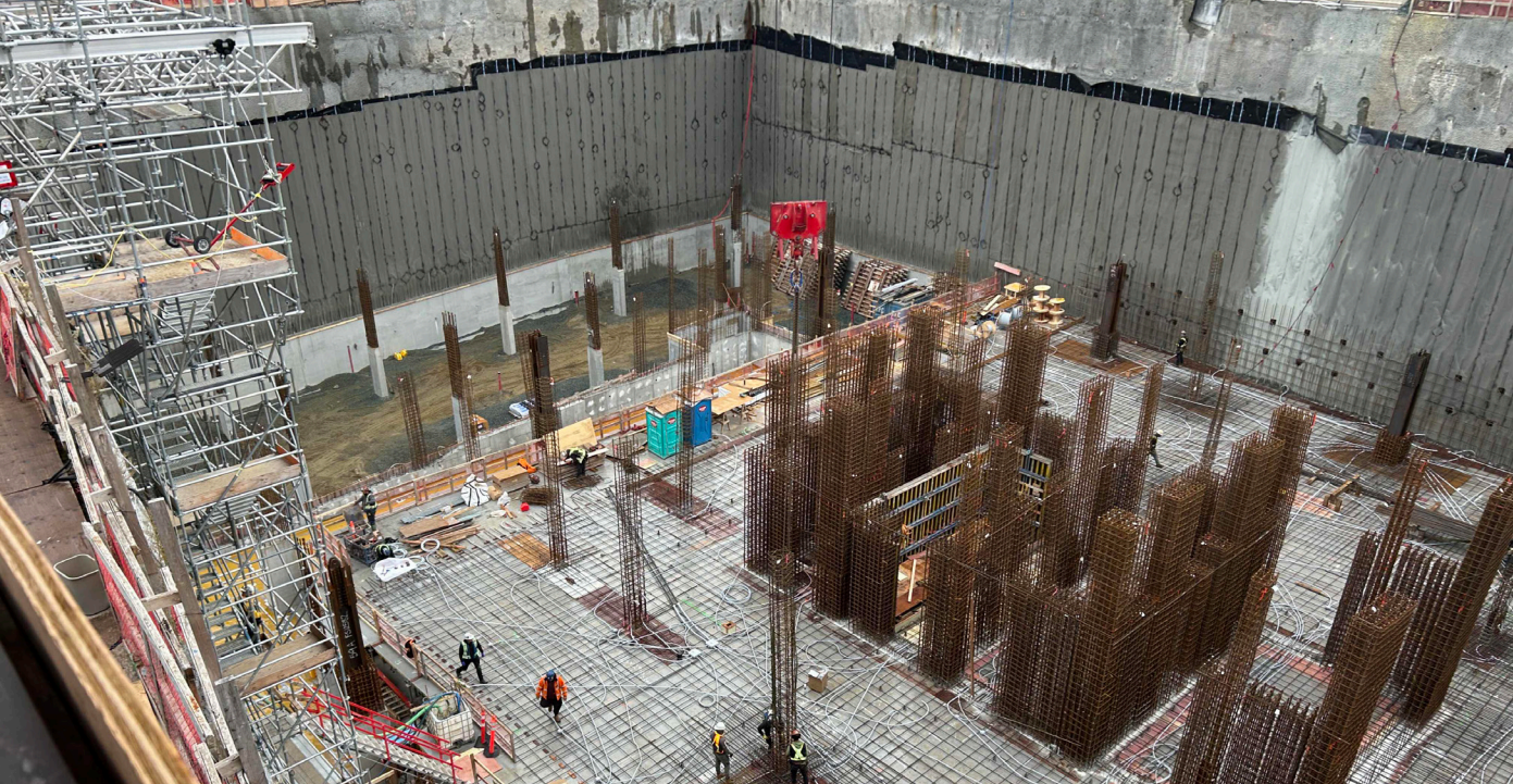
October 20, 2025: Formwork, rebar installation, and shoring activities underway.
