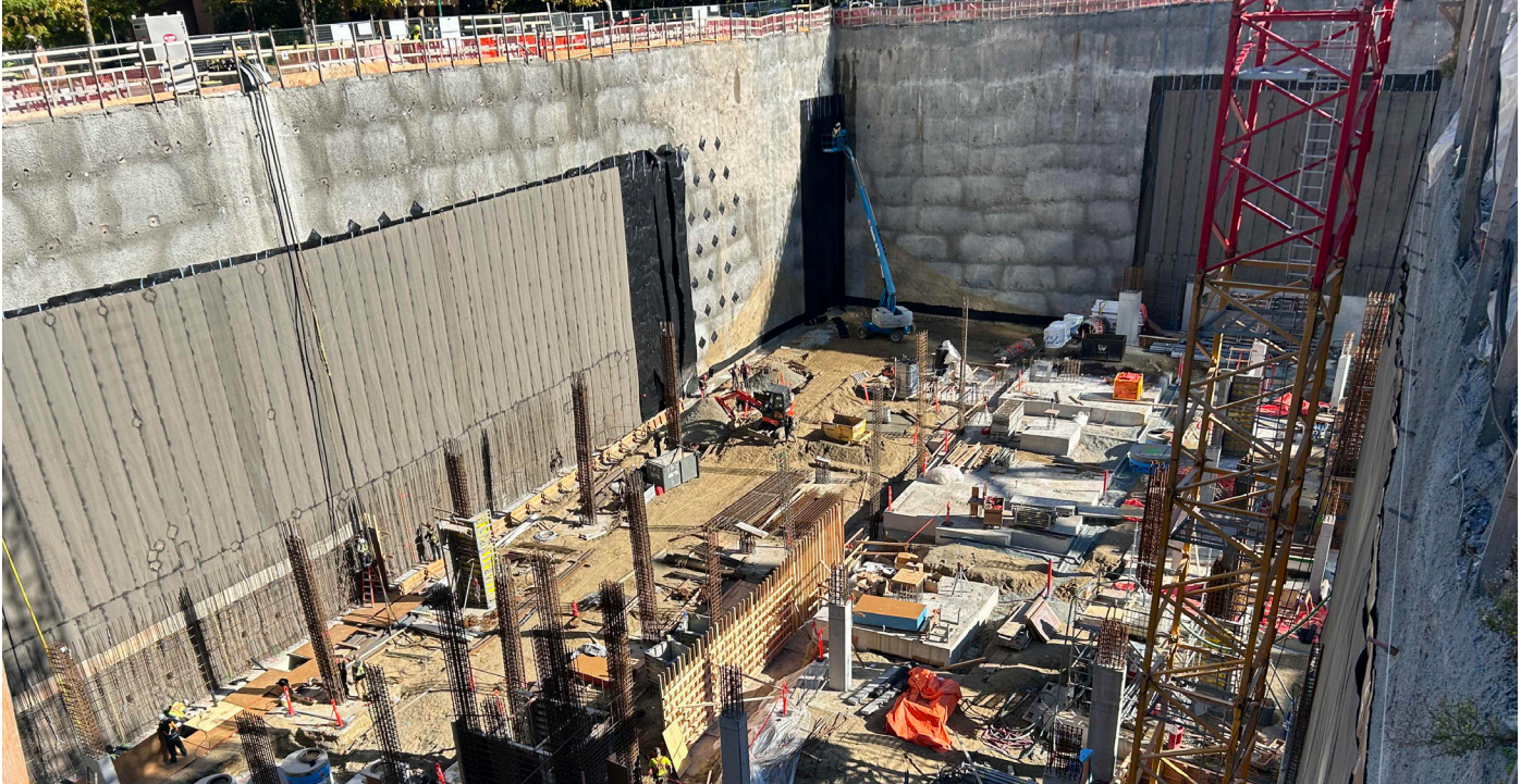
October 15, 2025: Northwest corner - vertical concrete work is ongoing.
