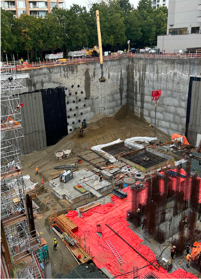
September 23, 2025: Progress on core footings ongoing.
