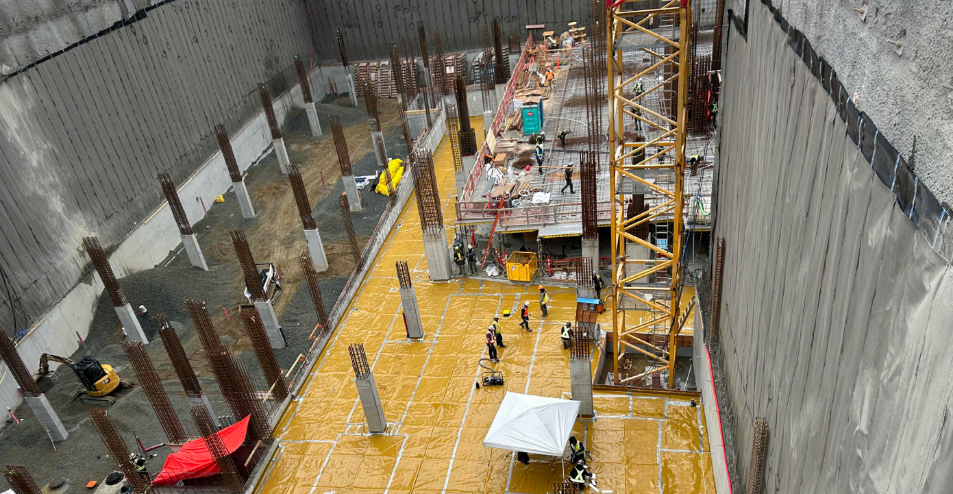
November 12, 2025: Slab on grade and vertical prep ongoing in northwest corner.
