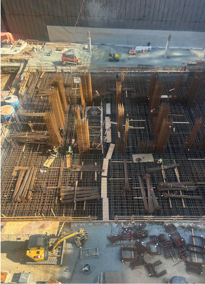
October 1, 2025: Footings prep ongoing.
